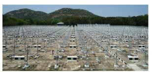
Figure 2. The antenna array and the TR modules, each feeding one antenna, of the MST radar.
